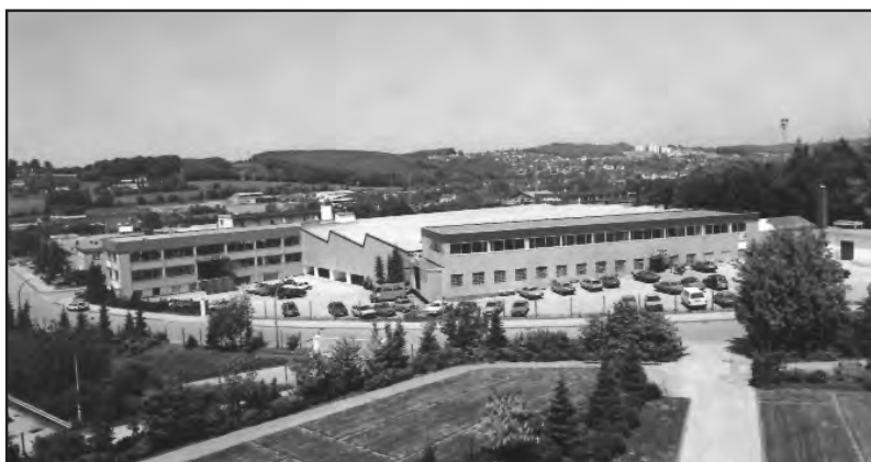
Fig. 1: RACO Engineering & Production Plant, Schwelm
