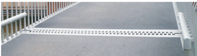
The comb profile between the segments in the area of pedestrians and cyclists!
