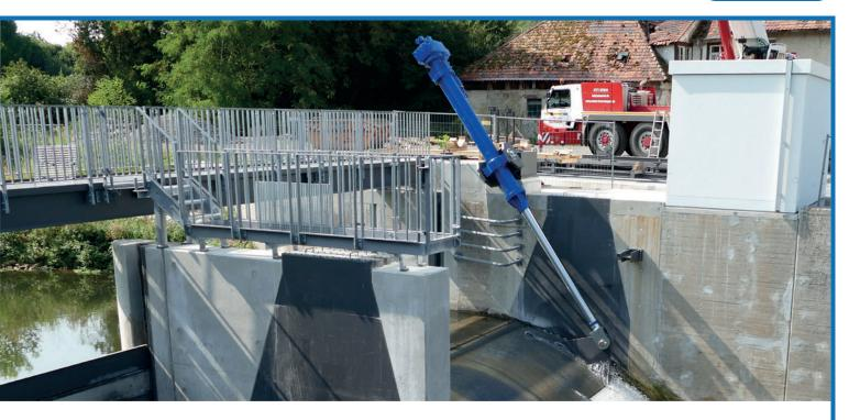
RACO electric actuators application in steel water construction - Weir flap actuation by means of electric cylinder with two integrated load measuring pins at the pivot pin reception.
